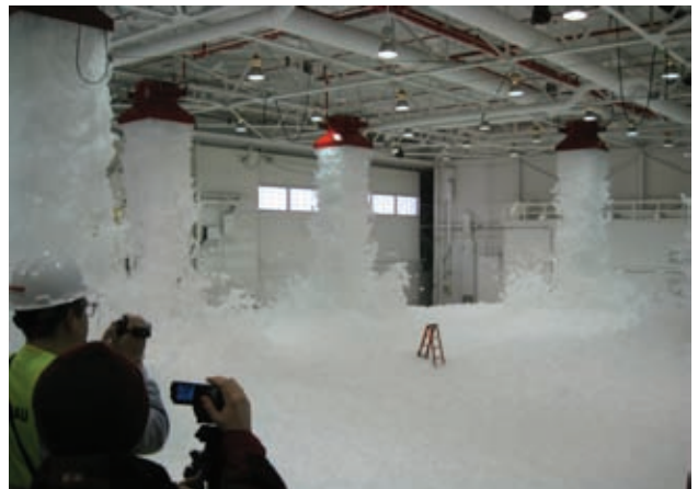
Figure 9 A variable-speed fire pump easily controls the design pressure at full flow when a foam system is operated and at no flow when the system is tested.
