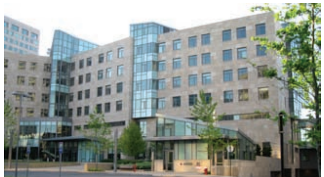
Figure 10 A variable-speed fire pump can help simplify complex fire protection systems for large institutions.
