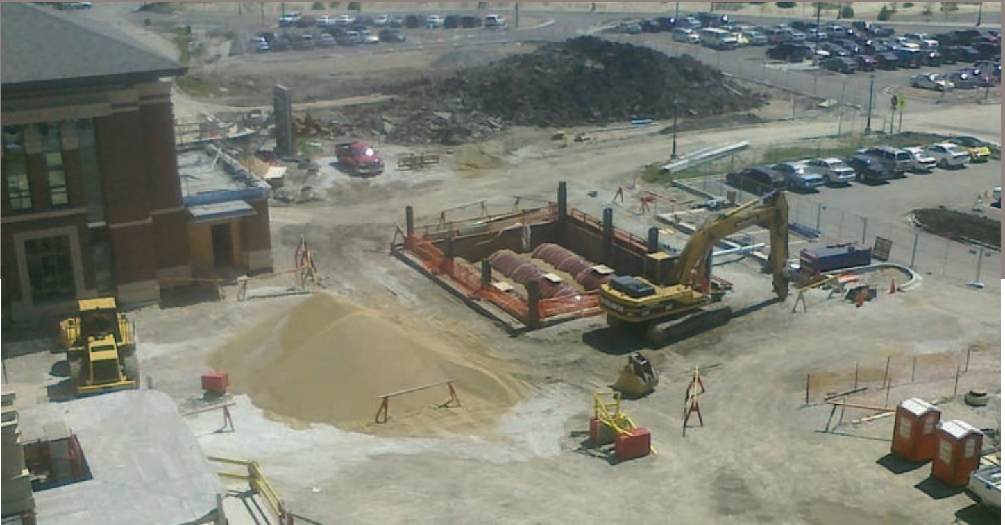
Figure 7 When buried storage tanks are required, using variable speed can quickly adjust the discharge pressure of the fire pump without cavitation.
